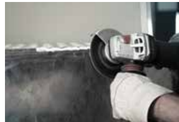
Removing welded seams
