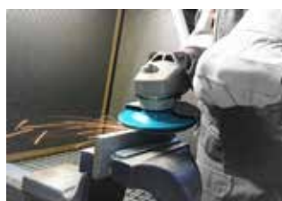
Weld seam preparation
